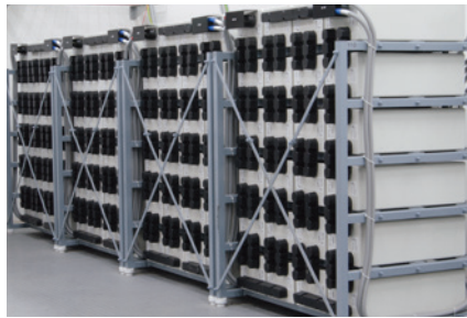
Energy Storage System
